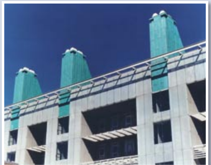
Cambridge University, Discharge Stack Enclosures
